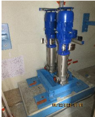
Installation of the demineralised water pump skid in the auxiliary building
