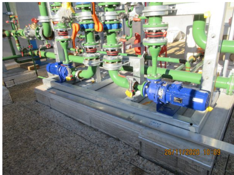
Auxiliary building (BMR) roof: ongoing installation phase
