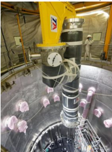
Lowering of the reactor vessel (also called reactor block) into the RER pool
