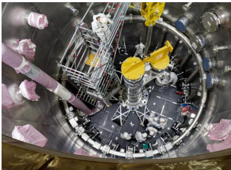
Installation of the vessel at the bottom of the reactor pool
