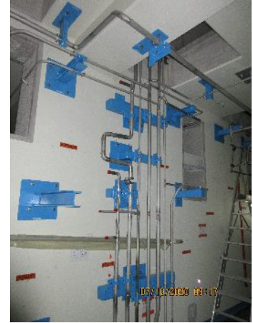
Installation of piping systems in the nuclear unit building (Level -2)
