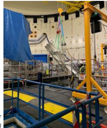
Installation of the floor frame in the JHR building
