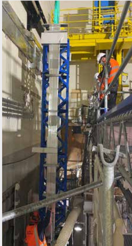
Installation of the gate frame
