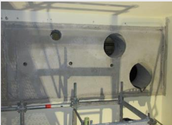
Creation of openings and preparation of these openings prior to the assembly of the HVAC and electrical systems in the reactor building
