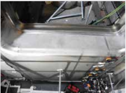
'Suitcase corner' lining completed
