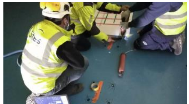
Drilling activities secured by steel detection using radar equipment
