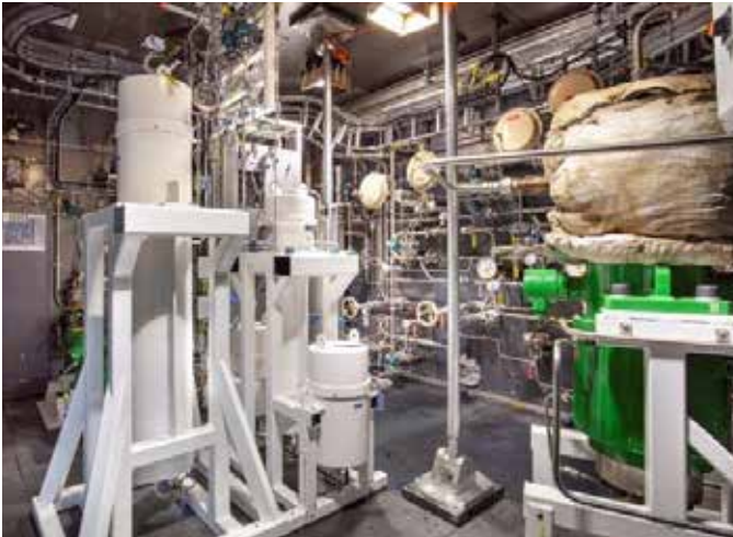
Overall view (purification filters in white)
