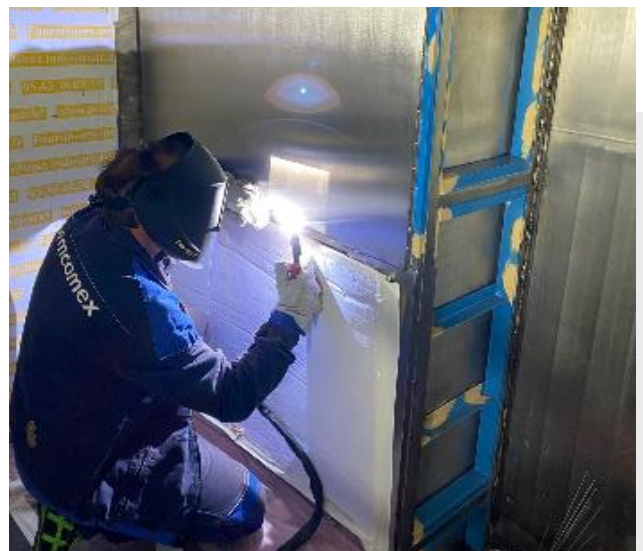
Shielded partitions in the sliding doors
