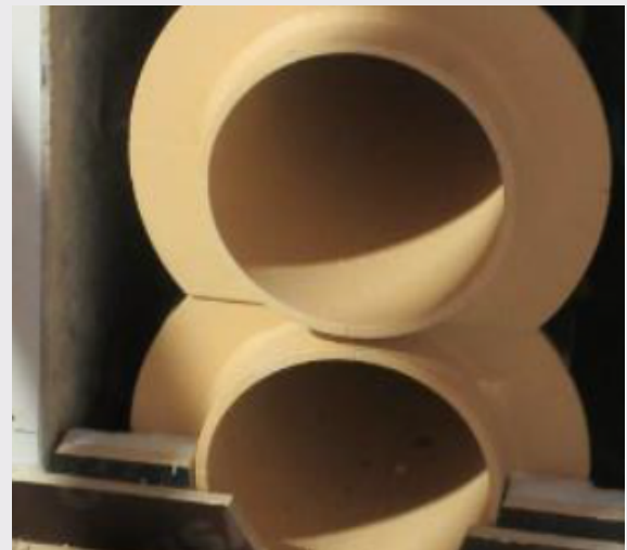
Creation of openings and preparation of these openings prior to the assembly of the HVAC and electrical systems in the reactor building
