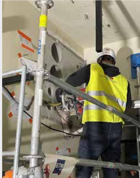
Creation of openings and preparation of these openings prior to the assembly of the HVAC and electrical systems in the reactor building
