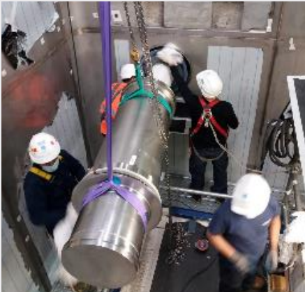
Assembly of EPI gamma penetration
