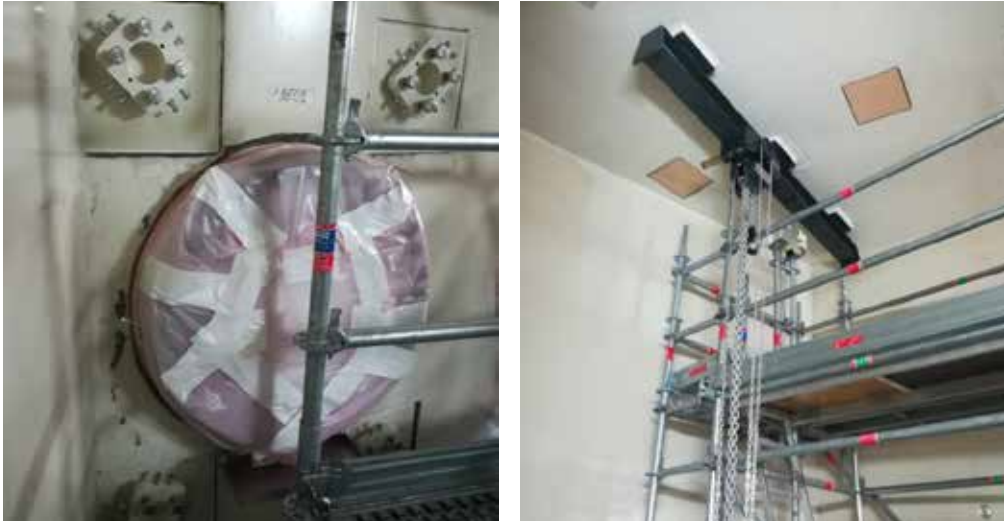
Installation of support structures and handling crane in the JHR
