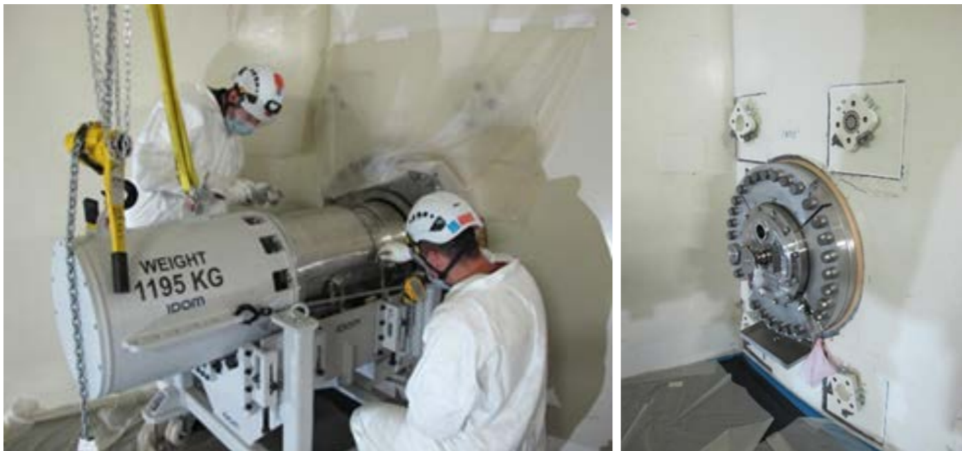
Collimator installation in the reactor pool feedthrough of the JHR
