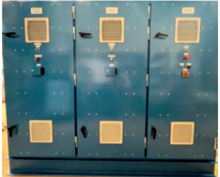
HVAC Electrical Distribution Panel
