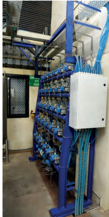
Transmitter rack of PPL-CLOE facility
