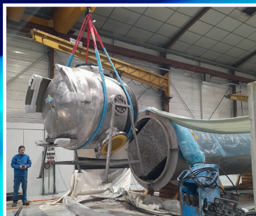
Cutting the heat exchangers
