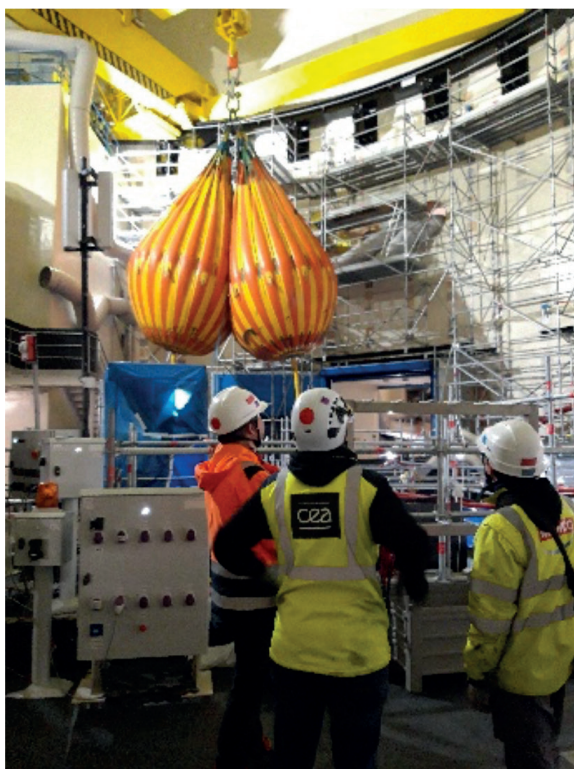
Polar crane re-qualification in the Reactor building Simulator room under construction in the BMX
