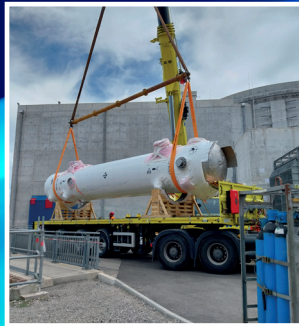
Removal of the heat exchangers
