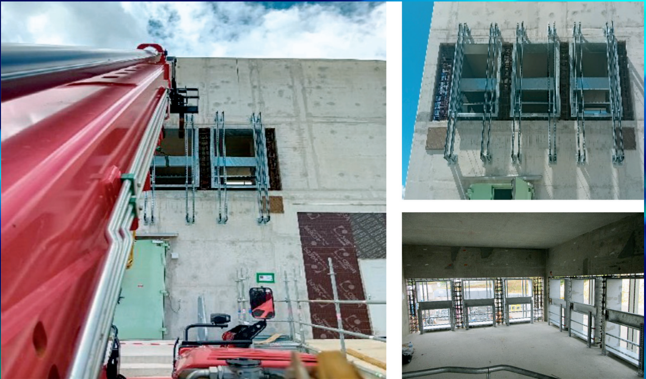
Installation of the pre-sealed inserts in BAS A and B
