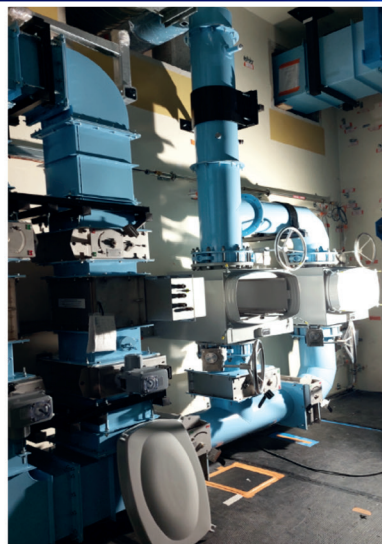
Installation of filter box and connectors
