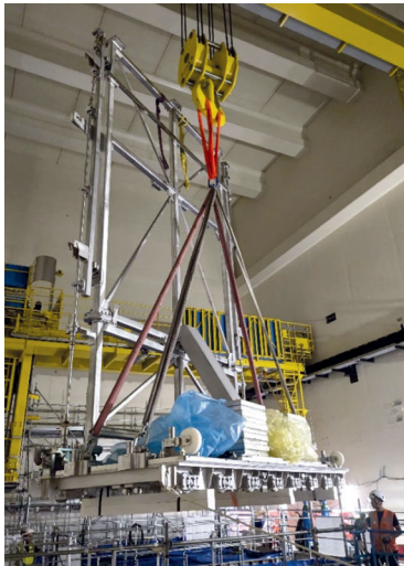
Delivery of a hot cell lifting unit
