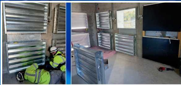
Installation of fresh air intake registers in BAS A and B
