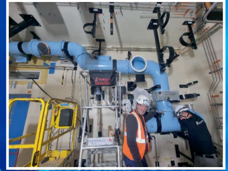
Installation of networks and equipment (terminal unit) at BUA
