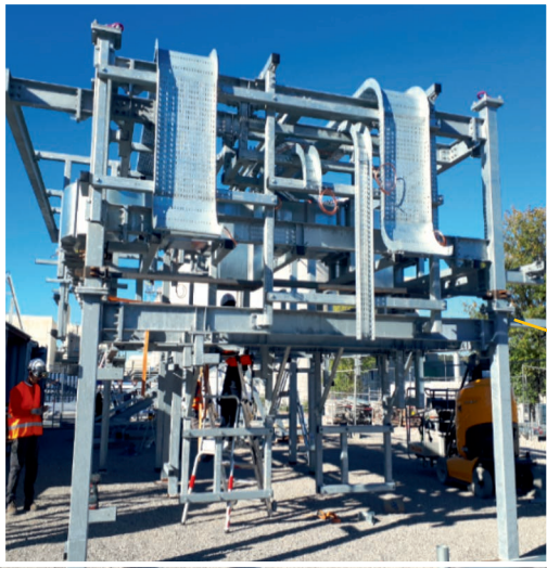
Assembly and installation of chassis module networks
