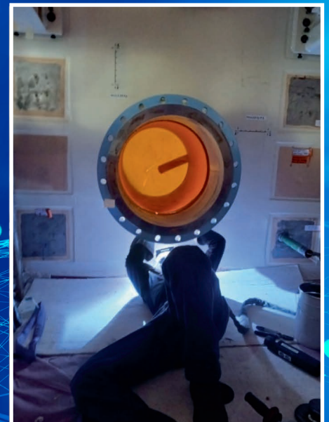
Assembly of penetrations
