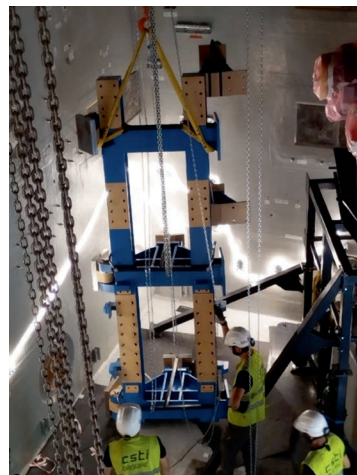
Second fixed points structure
