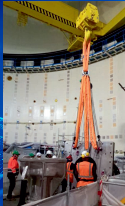
Handling of a pump volute and positioning in the cubicle
