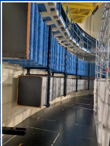
Installation of ducts in mezzanine
